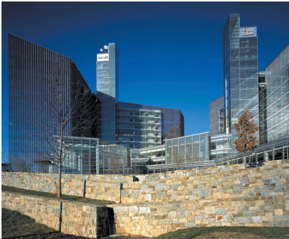
Although the Gannett/USA Today Headquarters in McLean, VA, is predominantly clad in glass, the landscaping features fieldstone walls of Carderock Stone from Tri-State Stone and Building Supply.
