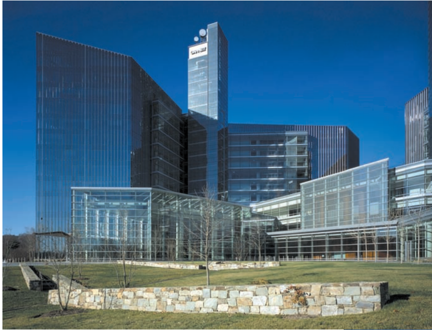
The fieldstone walls can be found throughout the building site, and they help connect the project to the earth.
